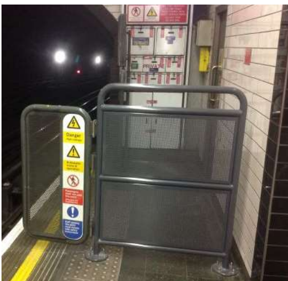
Marble Arch end of platform barrier and gate for Gateway.
